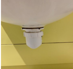
D: Wash basin in a supermarket – bottom end crevices of the waste water pipe showing accumulation of microbial biofilms. These are hard to reach areas with real risk of cross-contamination.
